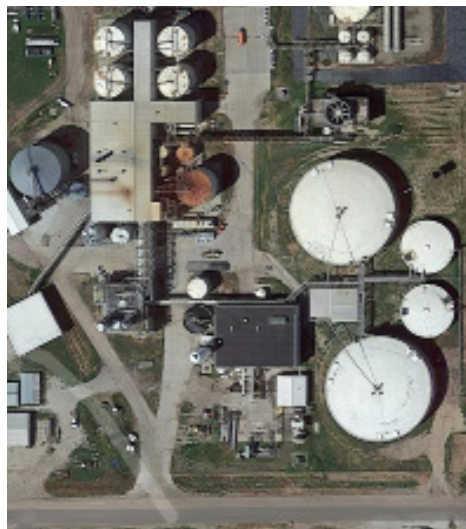
AltEn Methanol plant in Mead, NE
