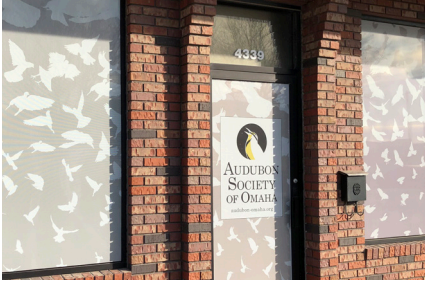
Strike-proof window films are now installed on large windows at the ASO's office.
